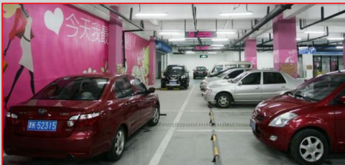
Covered car parking facility for each flat
